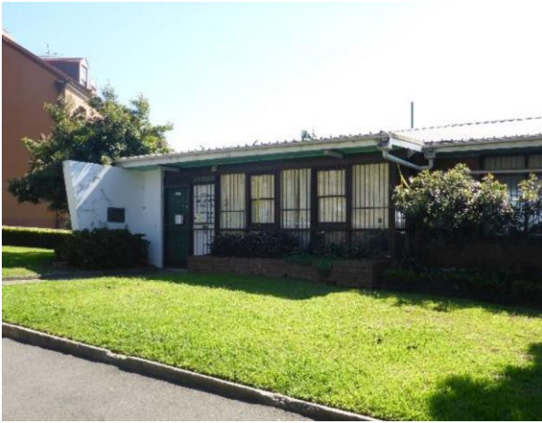
Picture 1 – Subject site from street frontage
